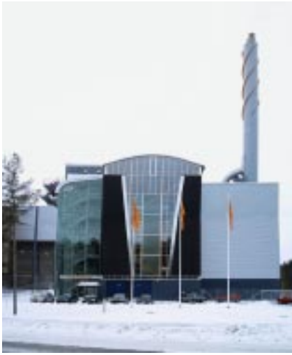
The main raw material in the biofuel heating plant in Turku is logging residues of a whitewood. Also other forest retreatment and mechanical forest industry by-products such as dust, shell, wood chips and cutter chips will be exploited. (Picture: Photo archive of Turku Energia, Esko Keski-Oja)
